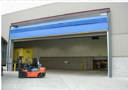
Monitoring Exterior for Motion
