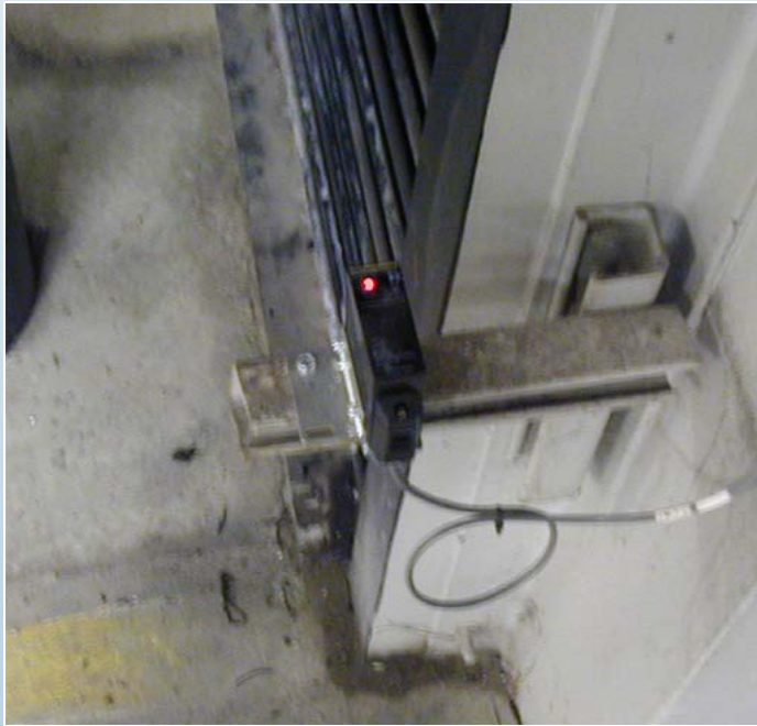
Photo-Eye & Door Reversing Edge Monitor Door Opening
